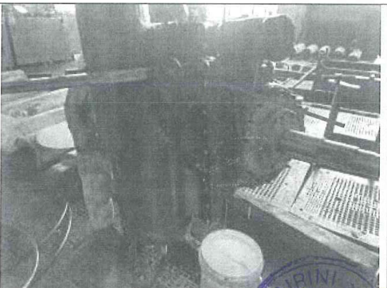
P6, The control valve had been test after renewed all the seal kit, it is in the good condition.
